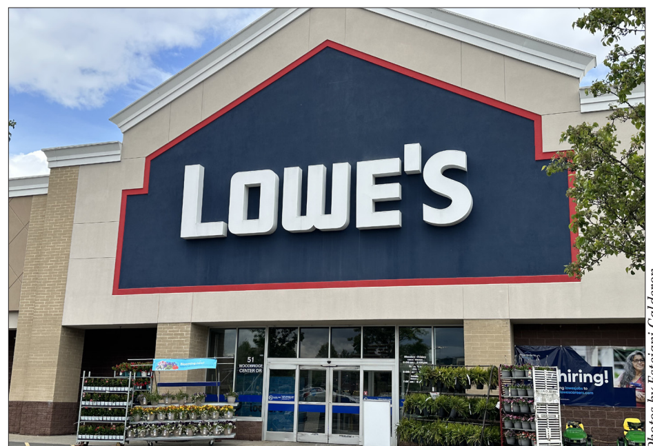
The outside of the Lowe's in Woodbridge
